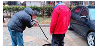
Special Initiative for Heating Water Loss Control
